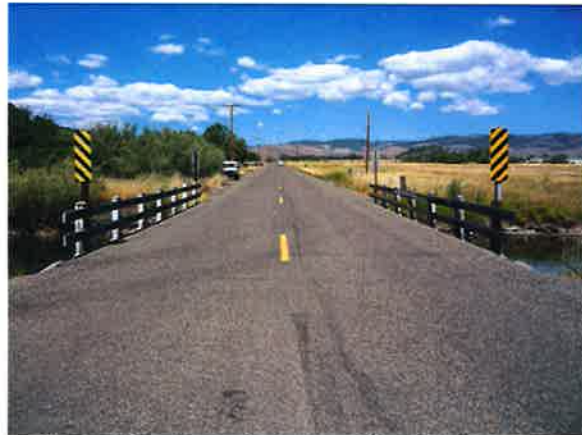
Cooke Canyon Rd looking north
