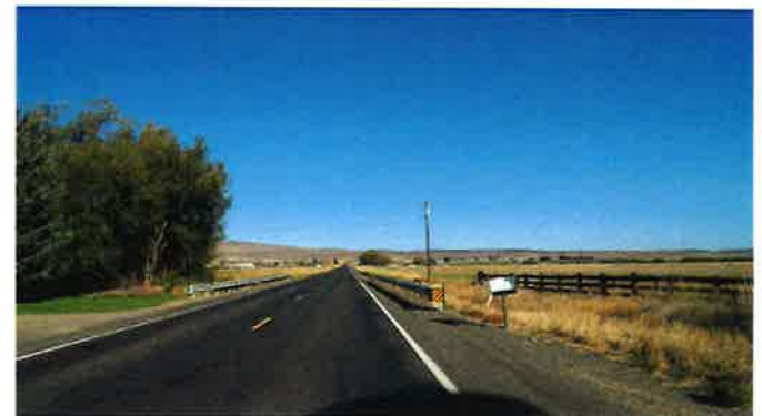
Vantage Hwy east of Parke Creek Rd
