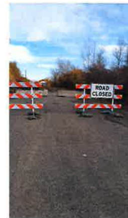
Bar 14 Rd with barricades after bridge removed
