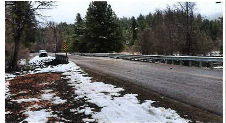
N.F. Teanaway Rd Bridge #16203-looking East
