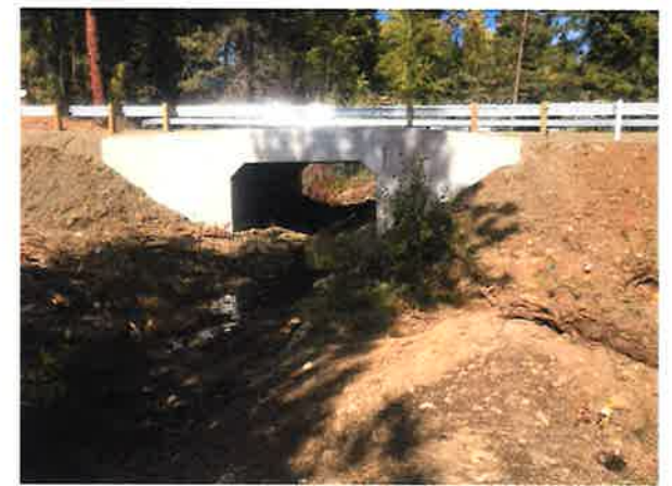
Storie Creek culvert finished in 2019
