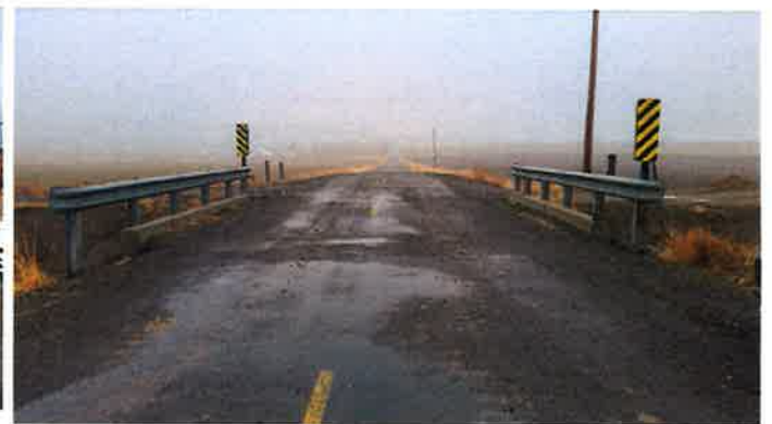
Bridge Rails to updated—4th Parallel Rd
