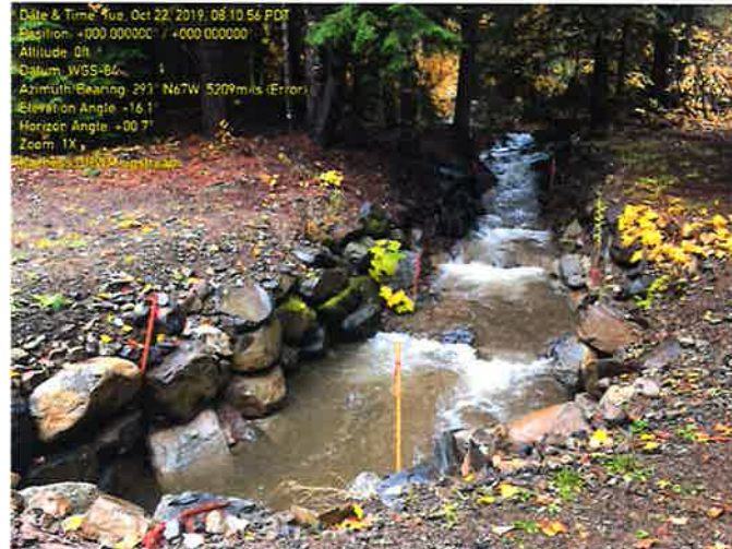
LOOKING UPSTREAM FROM CULVERT
