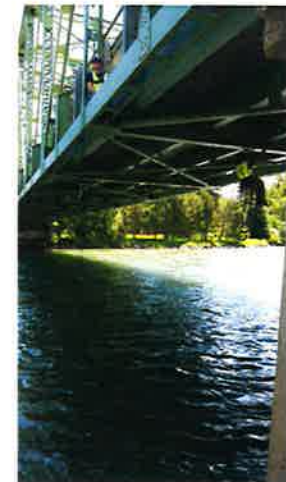
Under bridge during inspection
