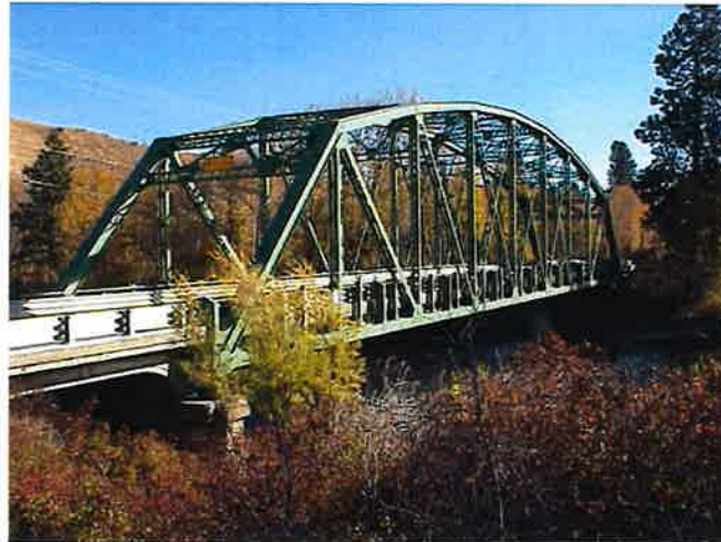
N. Thorp Hwy Bridge over Yakima River
