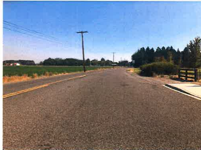
Sanders Rd-showing city sidewalk
