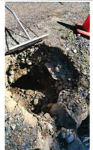
Undersized culvert
