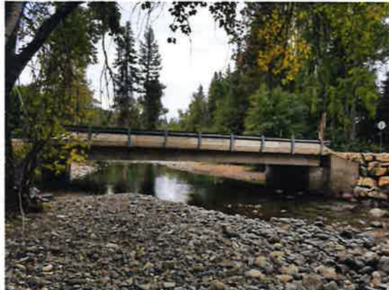
N.F. Teanaway Rd Bridge # 16203-looking South
